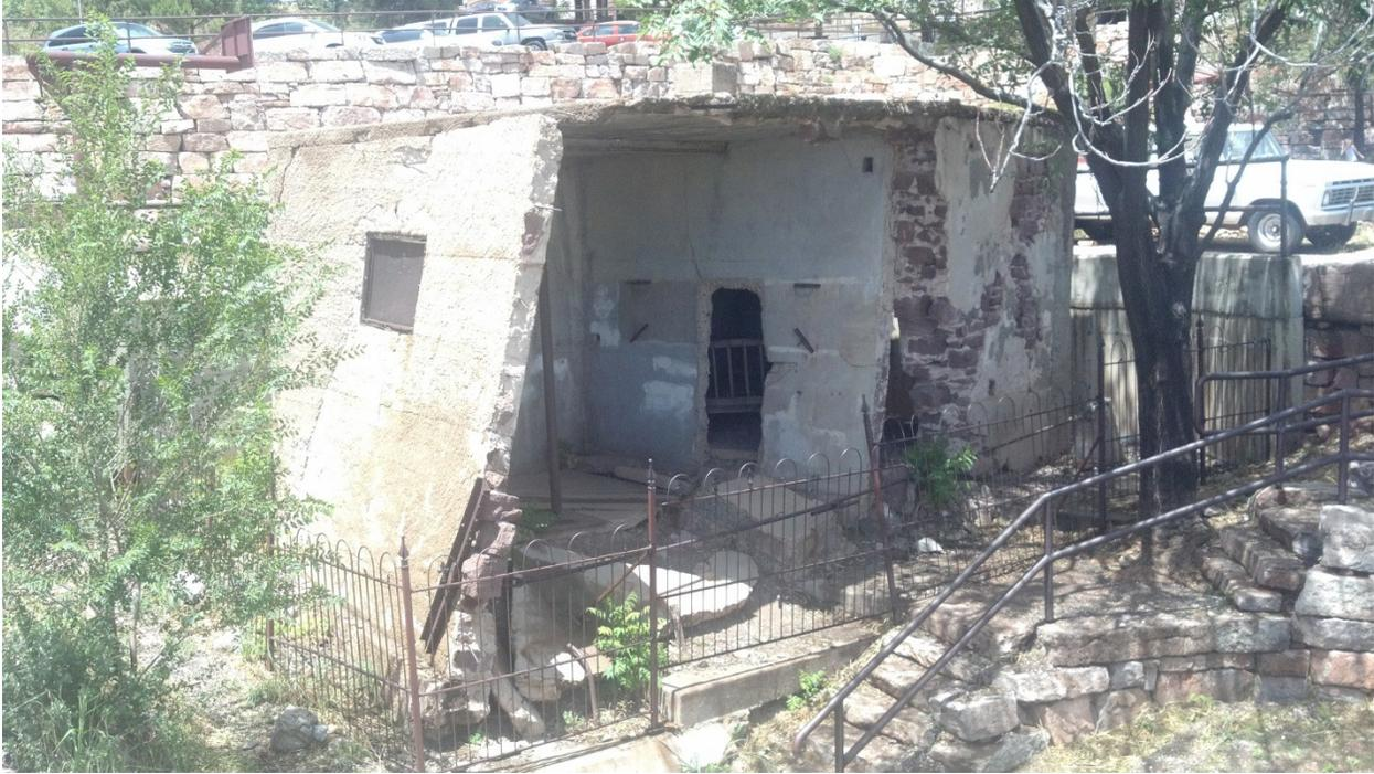
**Figure D1-9. Former Jerome city jail that was deformed by the 1936-37 Hull St. landslide.**
